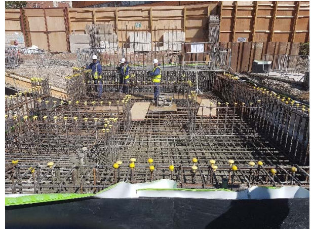
Concrete being poured to the main tower containing the central stair and lifts
