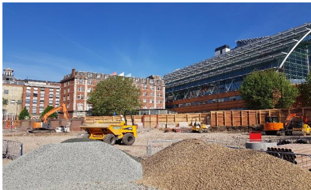
Ground preparation for the piling works
